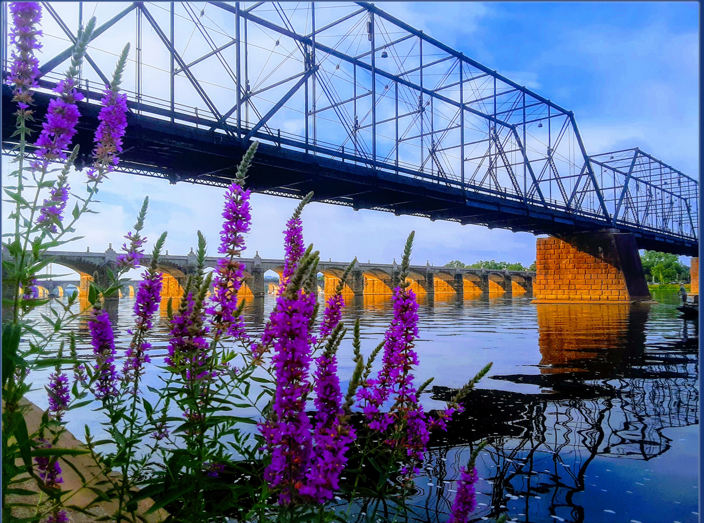
Historic Walnut Street Bridge
