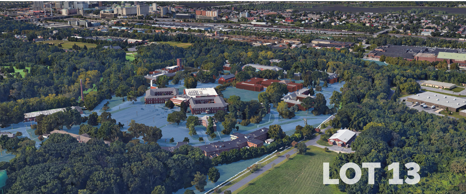
Aerial Images of the Four DGS Annex Property Lots
