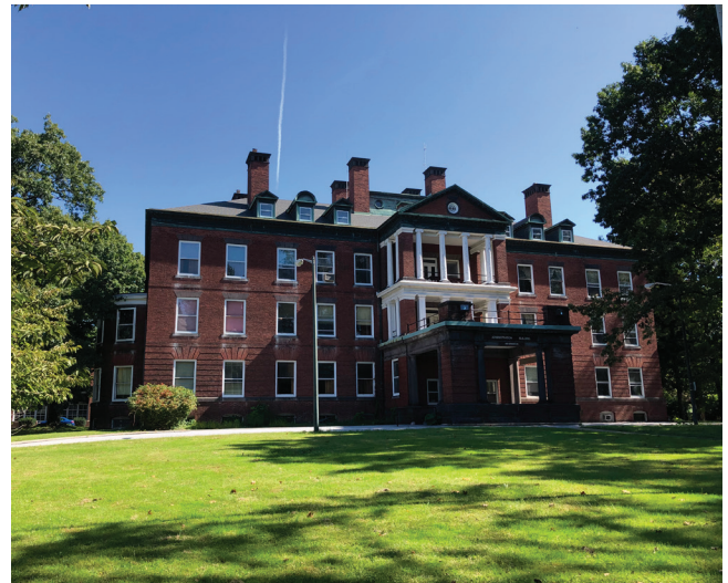
Admin Building, Main Entrance
